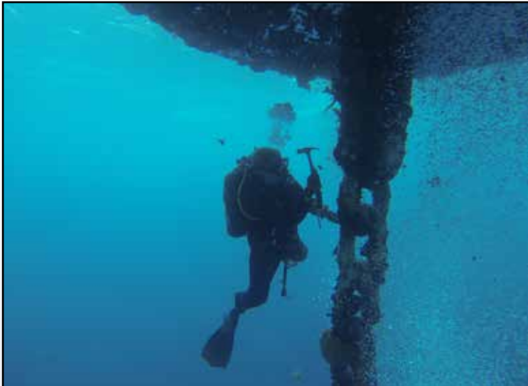
Lieutenant Nick Brown, from NAVFAC Engineering and Expeditionary Warfare Center, cleans a deep water mooring buoy during an inspection in Apra Harbor, Guam. (Photo by Construction Electrician Chief (SCW/MDV) Terence Juergens)
