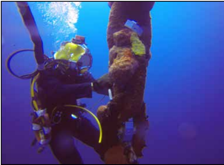
Builder 2 nd Class (SCW/DV) Joseph Hophan, from Underwater Construction Team (UCT) Two replaces zinc anodes on a deep water mooring in Apra Harbor, Guam. (Photo by Equipment Operator 1 st Class (SCW/DV) Manuel Terrero)
