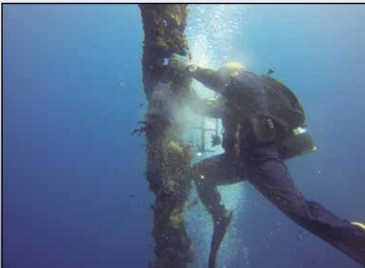
Equipment Operator 1 st Class SCW/DV) Manuel Torerro, from Underwater Construction Team (UCT) Two cleans a deep water mooring in Apra Harbor, Guam. (Photo by Construction Electrician Chief (SCW/MDV) Terence Juergens)
